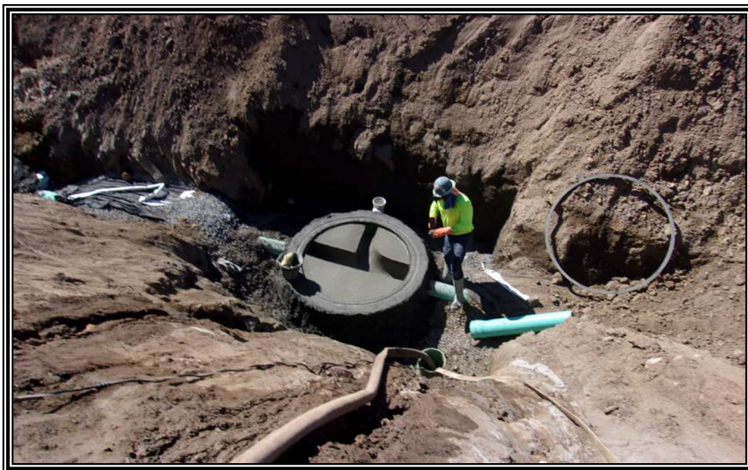
Base of sewer manhole in the Park Circle Development.
