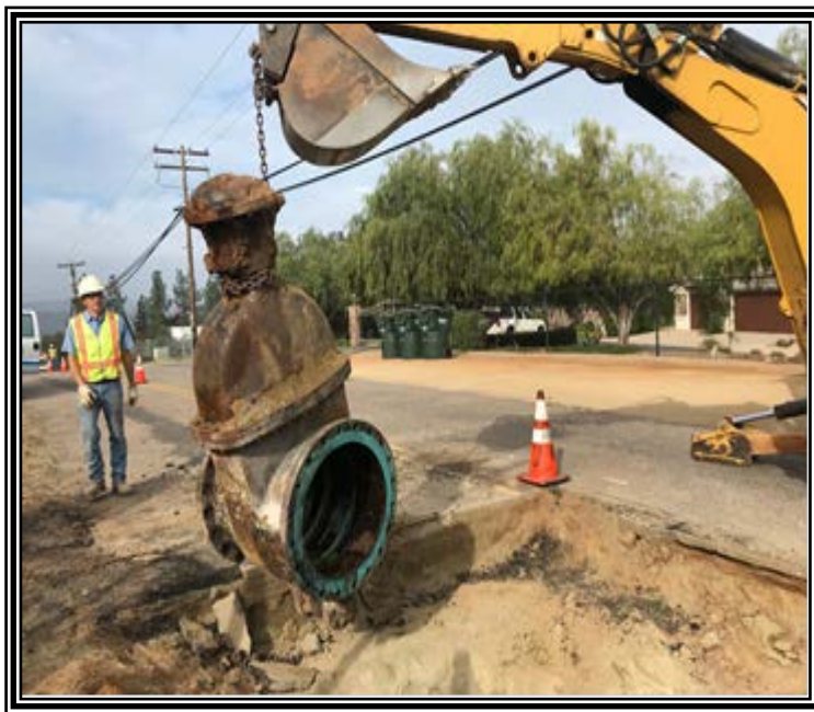
24-inch double-disk gate valve upgrade.
