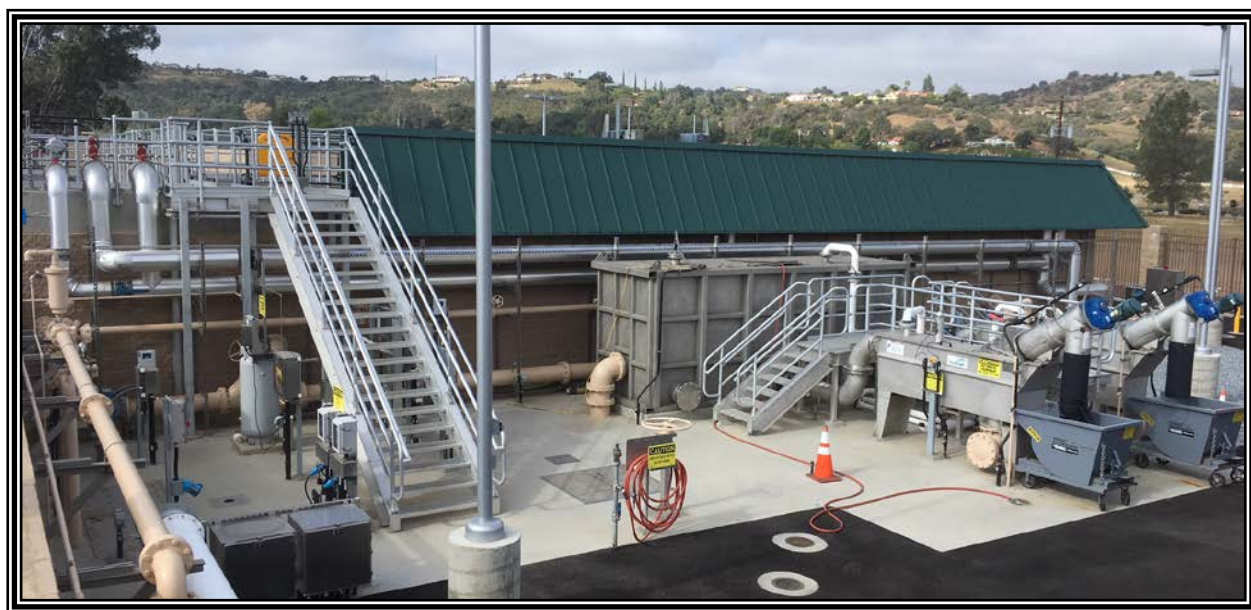
AeroMod Treatment Unit at the Woods Valley Ranch Water Reclamation Facility.
