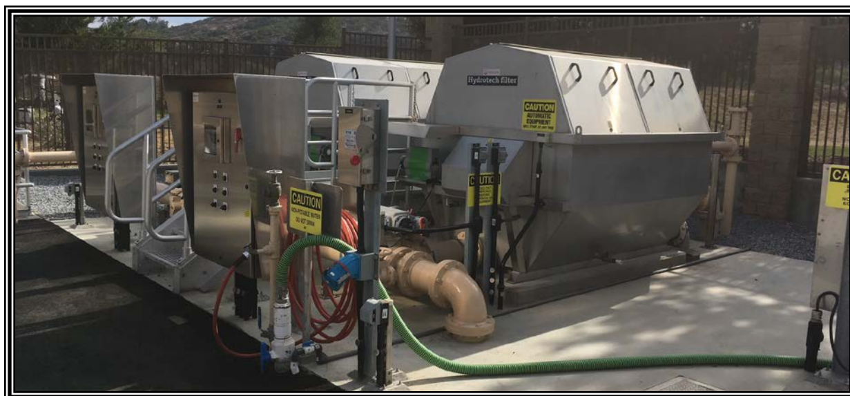
Woods Valley Ranch Water Reclamation Facility Disk Filtration System.
