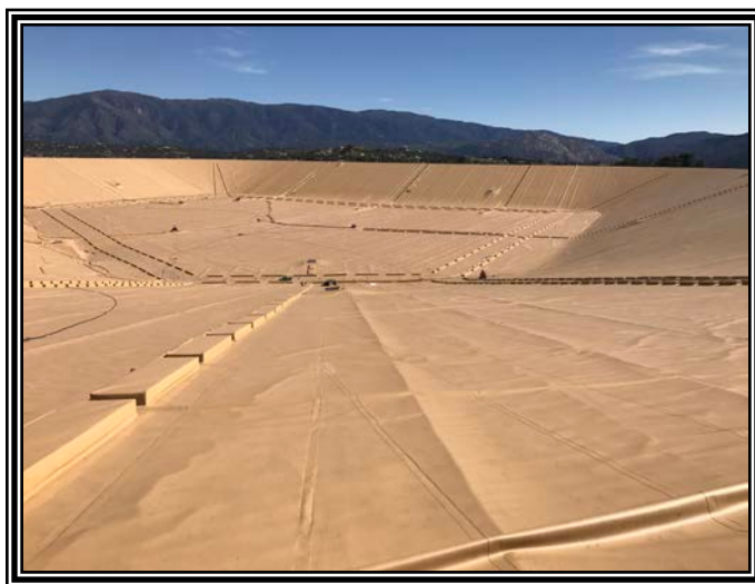
Cool Valley Reservoir Cover/Liner Replacement
