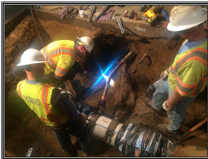
Leak repair at Old Castle.
