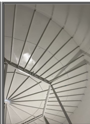
Interior Paint & Coat of McNally Reservoir
