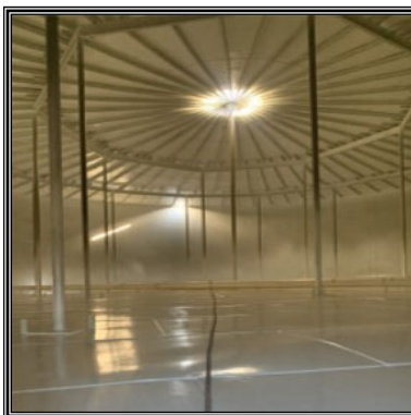
Interior Paint & Coat of Weaver Reservoir
