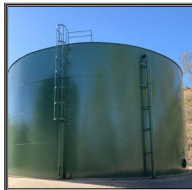
Exterior Paint & Coat of Burnt Mtn Reservoir
