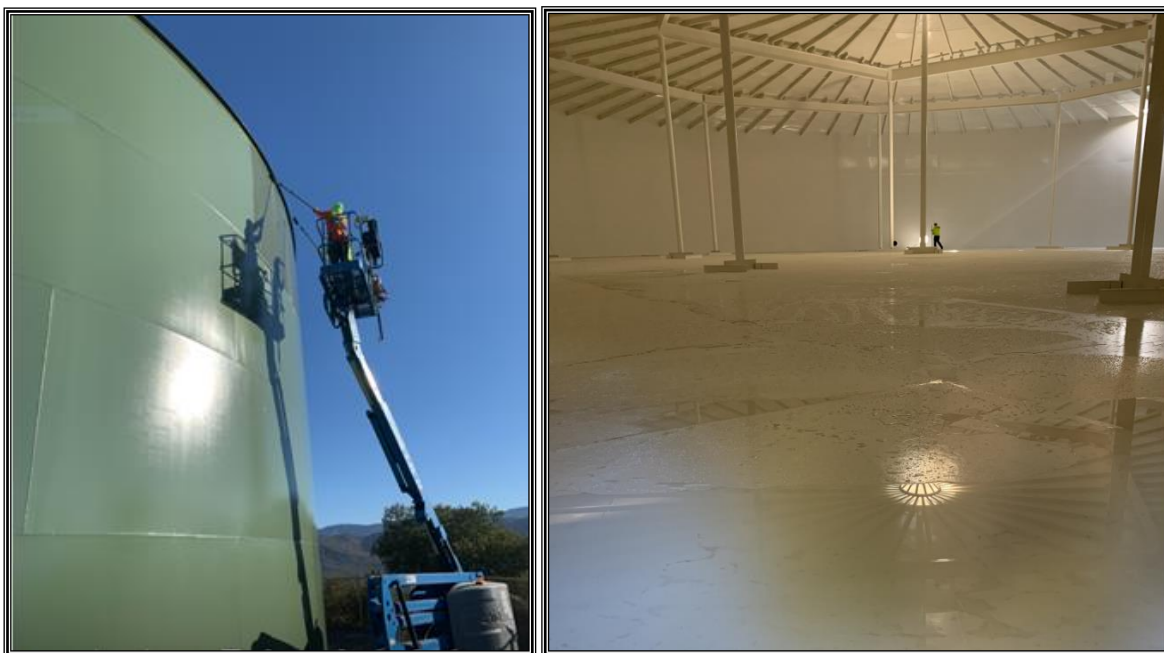
West Bear Ridge Reservoir Recoating and Painting of the exterior and interior.
