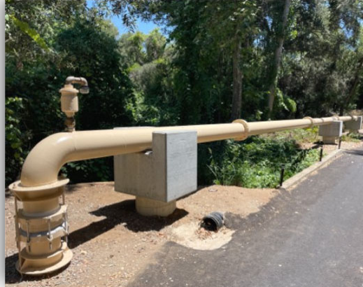
14-inch Pipeline Replacement – Creek Crossing.
