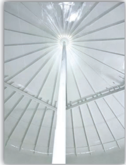
Interior Paint and Recoat of the Meadows No. 1 Reservoir.
