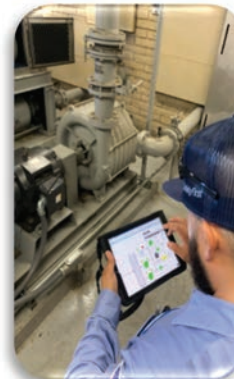
District staff using the handheld remote system at the Lower Moosa Canyon Wastewater Facility resulting from the recently completed SCADA upgrades and HMI Migration programming project.
