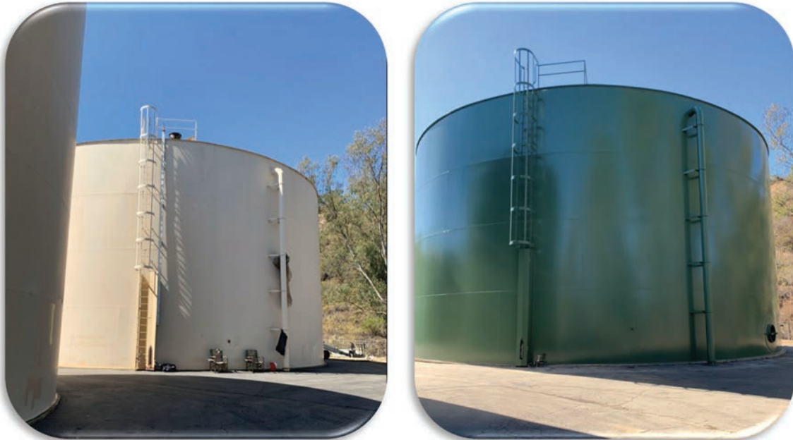
Before and after of the Reidy Canyon No. 1 Reservoir exterior Paint and Recoat.
