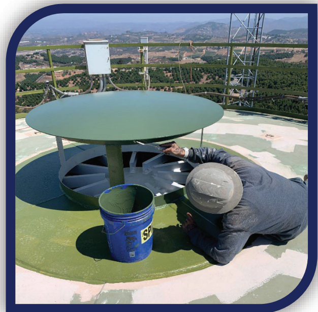
Circle R Reservoir Exterior Coating application.
