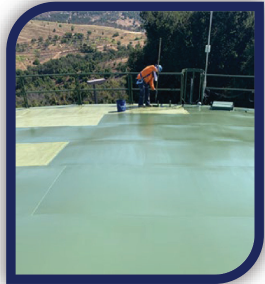
Application of exterior roof coating at Couser Reservoir.
