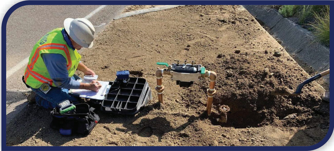
District Staff installing Advanced Metering Infrastructure (AMI) upgrade.
