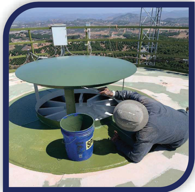
Circle R Reservoir Exterior Coating application.
