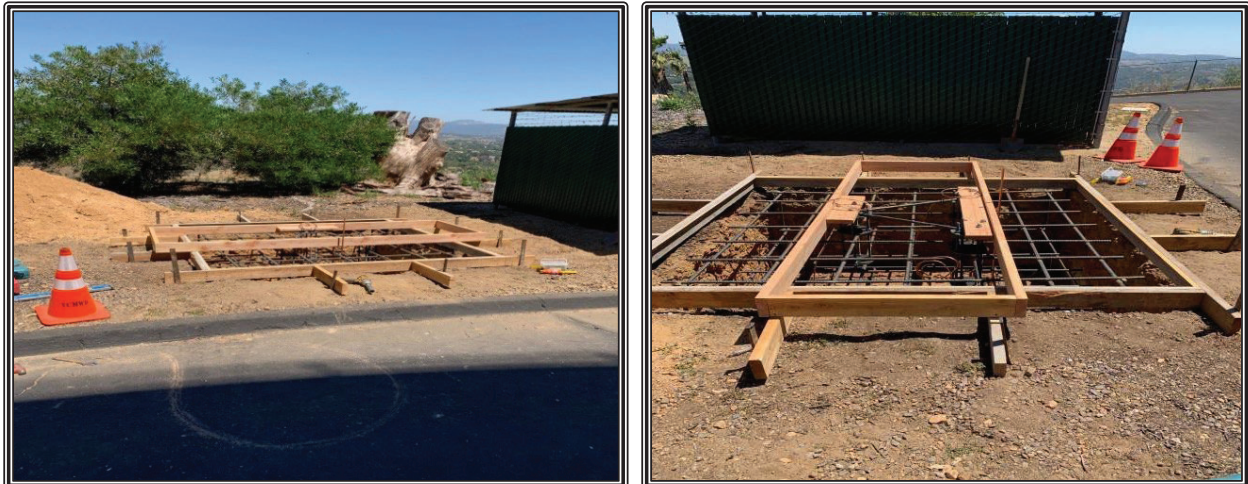
Construction of antenna base structure at the McNally Reservoir site for the Advanced Metering Infrastructure System.
