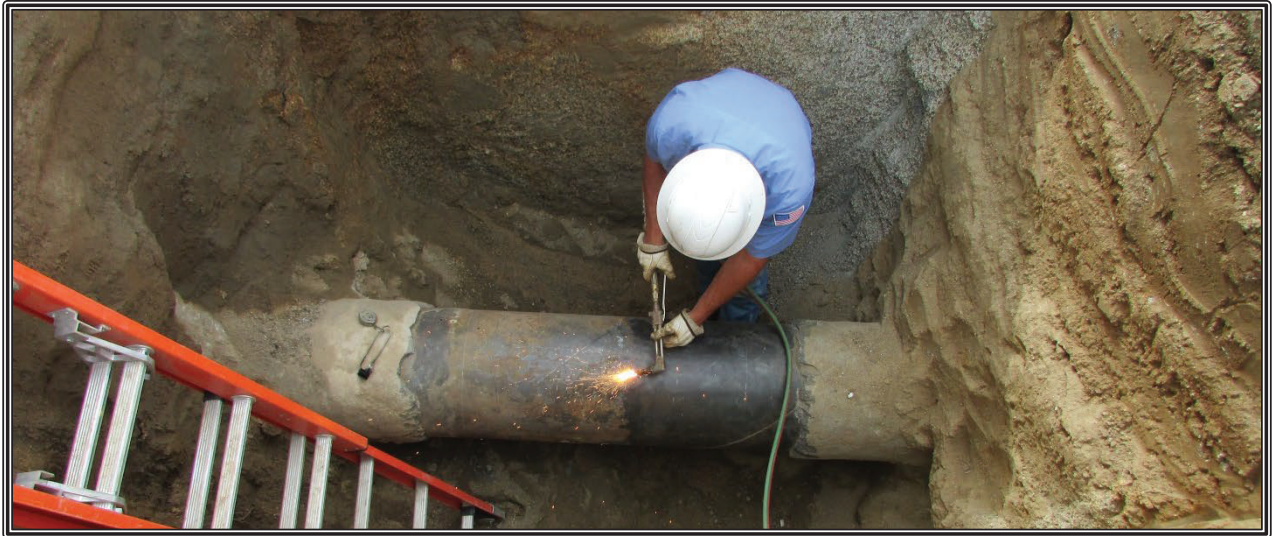
New valve installation on a 16" mainline.
