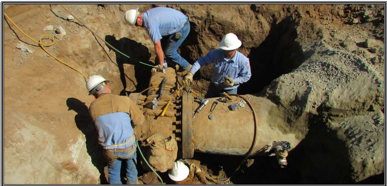
24" Valve Repair at Betworth Forebay Pump Station.
