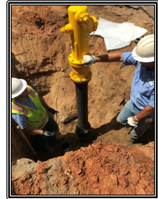
Fire Hydrant repair.
